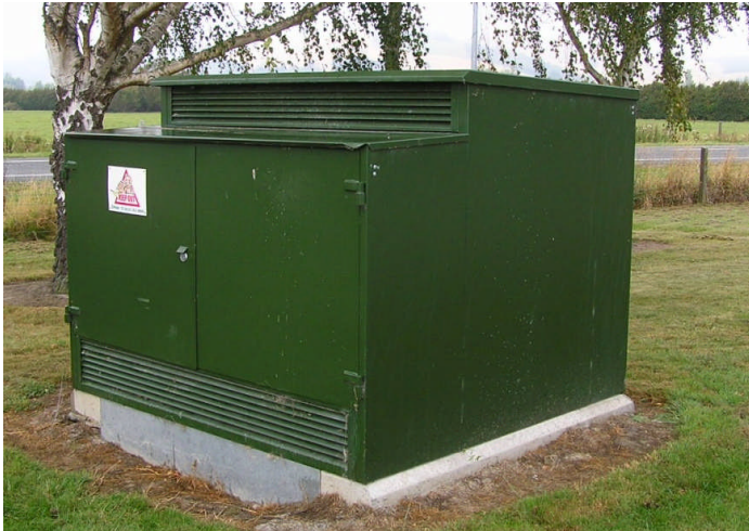
Figure 13: Example of a Concrete/Steel Kiosk
