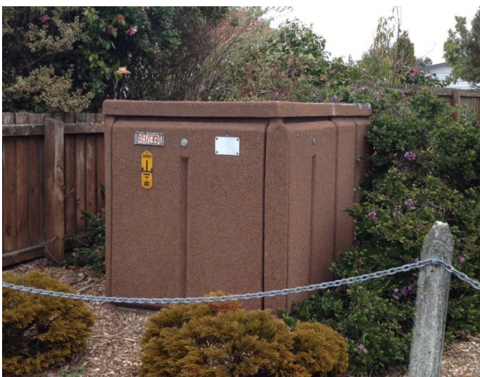
Figure 14: Example of a Fibreglass Kiosk
