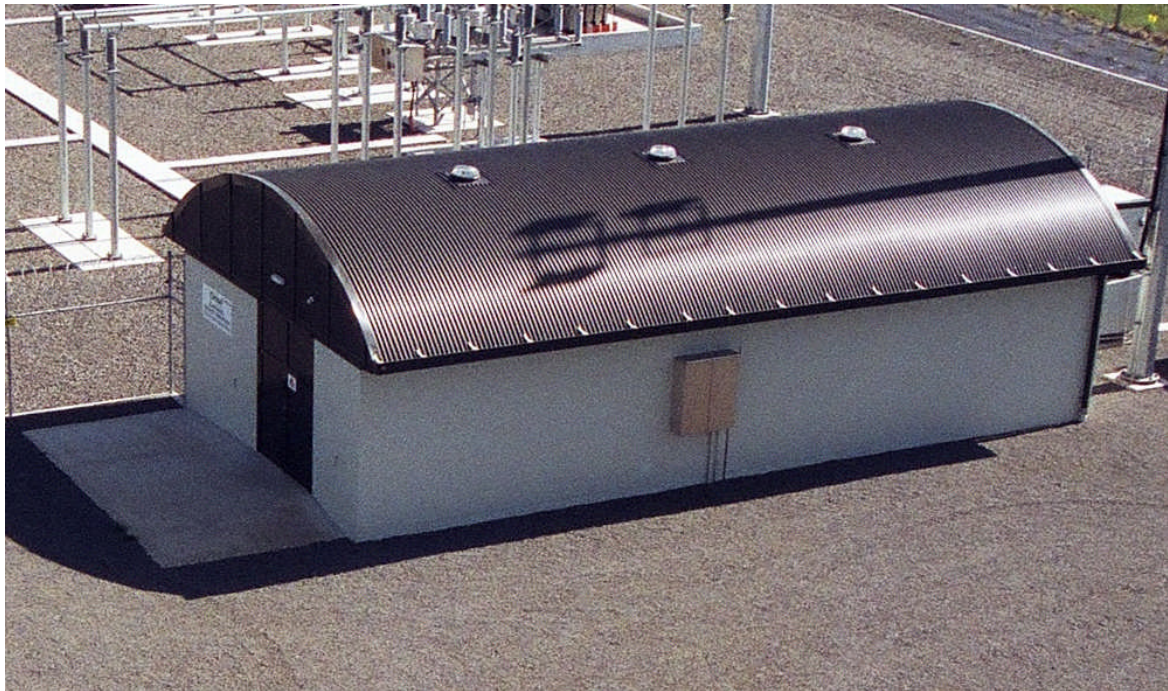
Figure 5: Concrete Block Construction – Dunsandel Zone Substation (2008)
