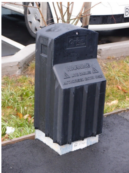
Figure 5b: Distribution Box – Current Design
