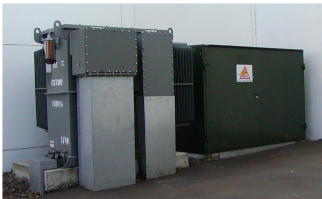
Figure 8: Typical Outdoor Distribution Substation
