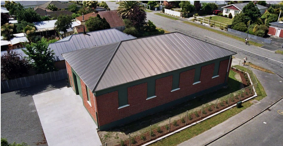
Figure 5: Grimseys Winters 11kV Zone Substation
