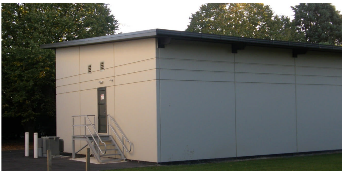
Figure 4: Concrete Tilt Slab Construction – Papanui Zone Substation (2010)
