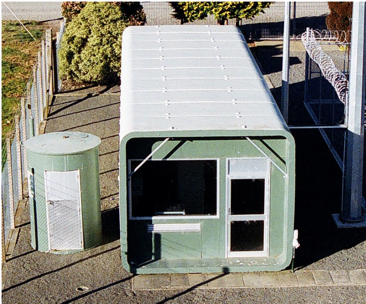
Figure 3: Modular Concrete Construction – Bankside Zone Substation (1983)
