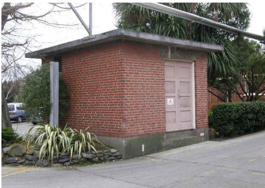
Figure 9: Example of a Privately Owned Distribution Substation – Davis Gelatine
