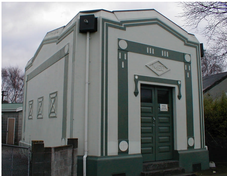
Figure 6: Network Substation (Built in 1930s)
