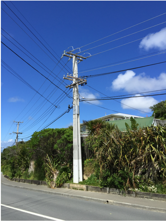
Re-conductoring for worst feeder programme, Johnsonville area
