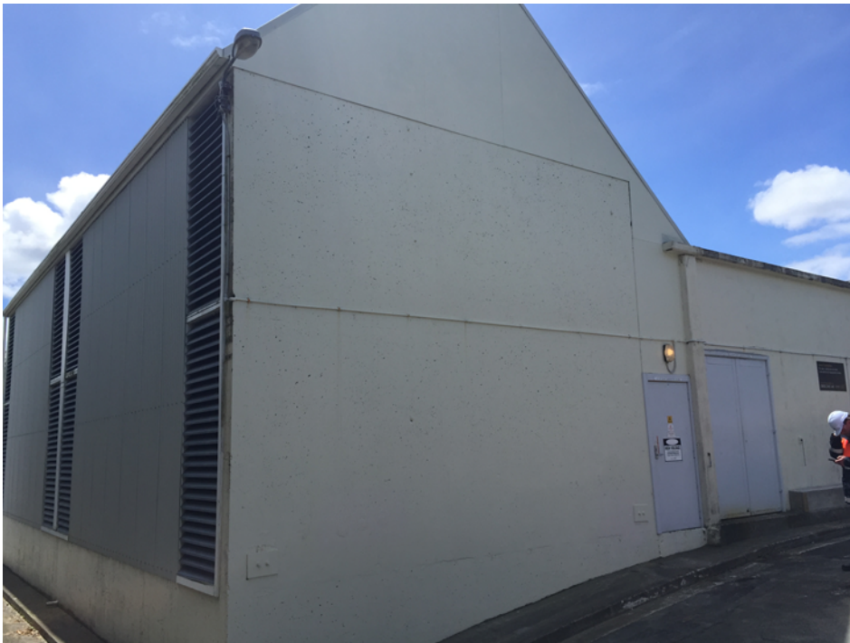
Karori substation showing substation extension for transformers on LHS, and seismic strengthening (exposed concrete block) added to base of existing building on RHS.
