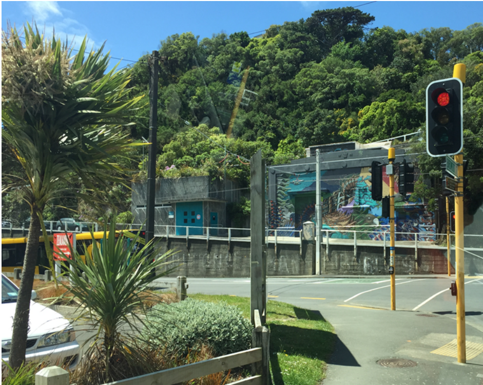
Example of substation built in 1925
