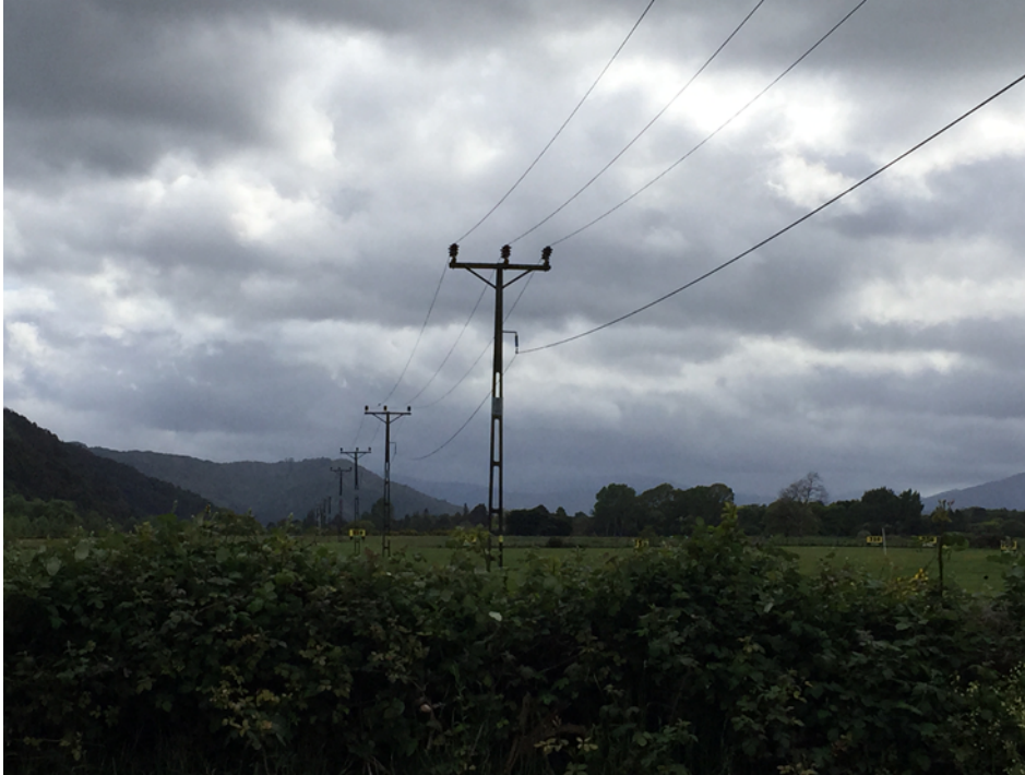
Example of older style concrete pole line across private property facing north. Recent line outages as a result of wind borne debris
