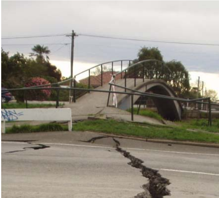
Earthquake damage to a walk bridge nearby to 66kV cable bridge
