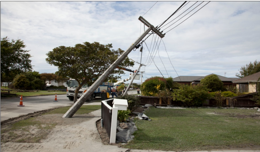
Poles also moved due to lateral spread
