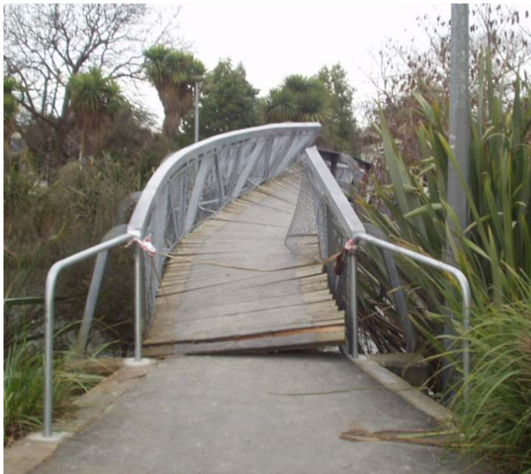
Earthquake damage to a walk bridge nearby to 66kV cable bridge
