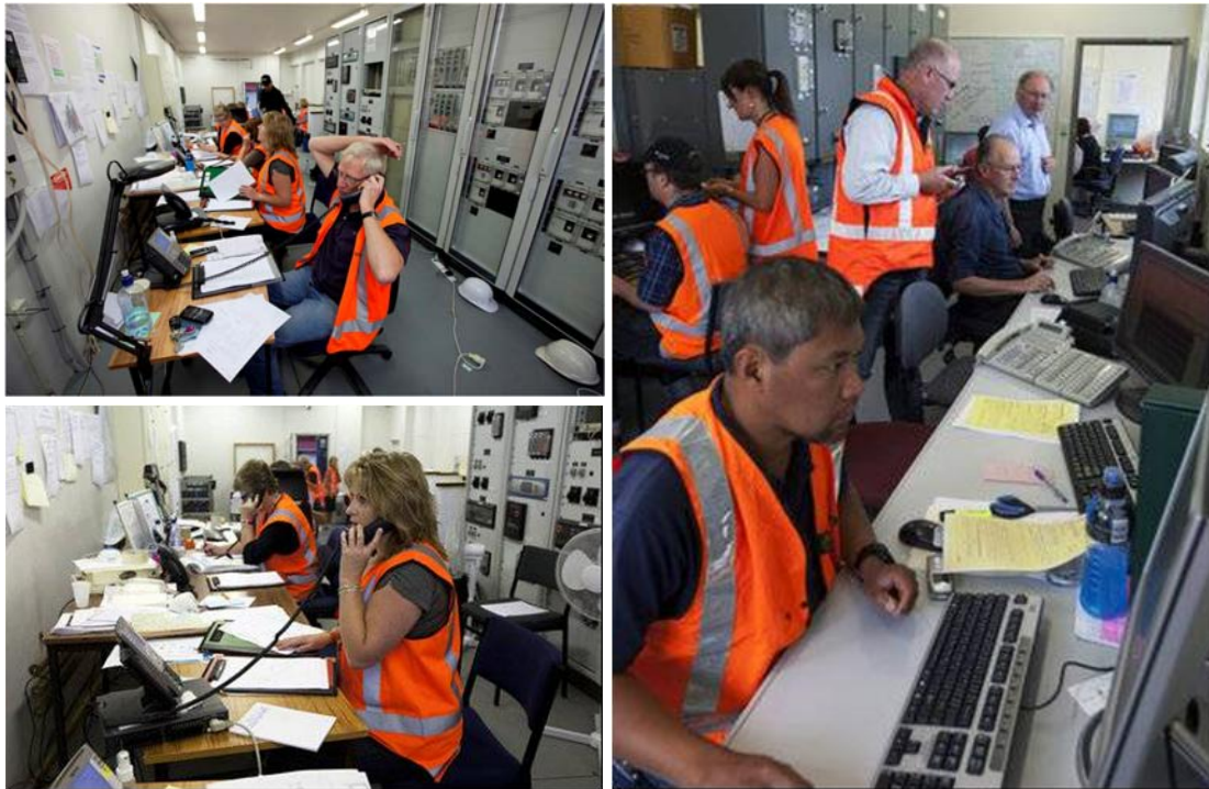
Our temporary (hot site) control room – February 2011
