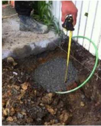
Figure 4: Work required to install a lateral and microduct in handhole
