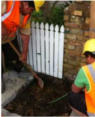
Figure 4: Work required to install a lateral and microduct in handhole
