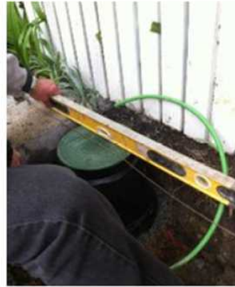
Figure 4: Work required to install a lateral and microduct in handhole
