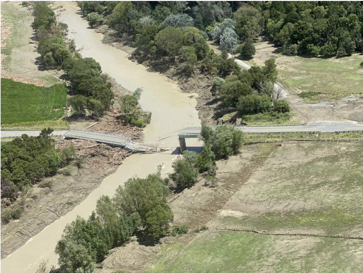
Hikuwai Bridge on the state highway linking Tokomaru Bay to Gisborne.
