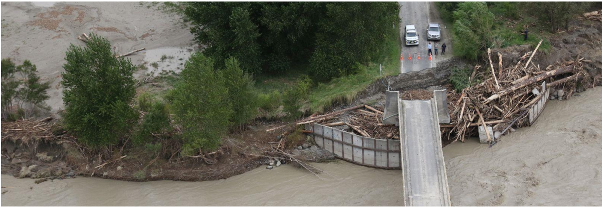
Image source: https://www.gdc.govt.nz/services/tairawhiti-road-to-recovery/flood-damaged-road-network
