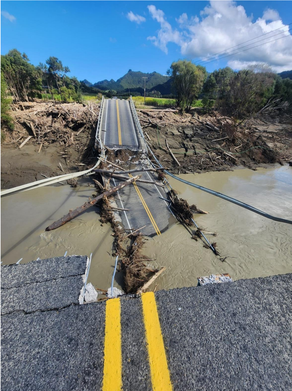
Hikuwai Bridge No.1 on SH35 isolated access to the coast
