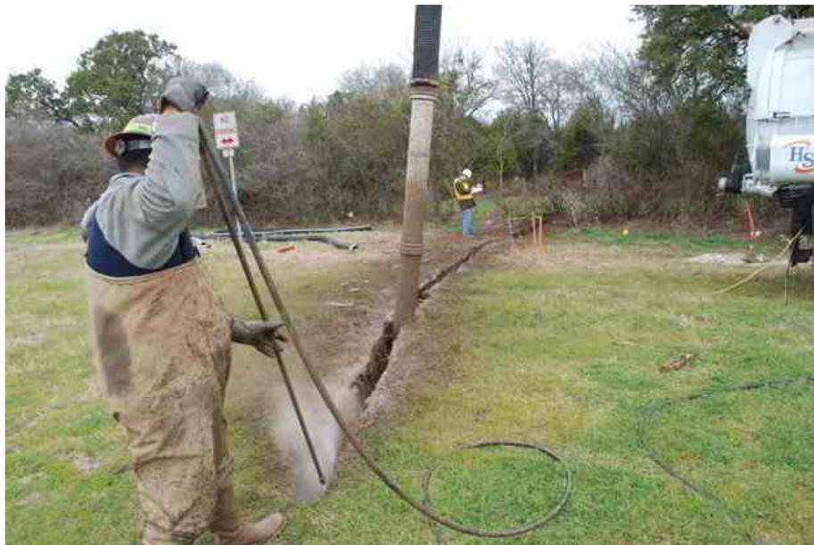
Sometimes called hydro trenching or hydro vacuum excavation, this technology uses high pressure water jets to loosen the soil within the trench producing a watery slurry which is then removed using suction from powerful vacuum equipment. The use of water helps reduce the soil's holding strength thus helping to break the soil and suction them easily. When excavating frozen ground, hot water can be used to thaw the frozen ground and dig through.
