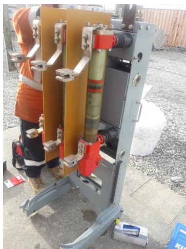
Figure 8.59: Indoor minimum oil-filled circuit breakers (left) installed in 'outdoor cubicles' (right)
