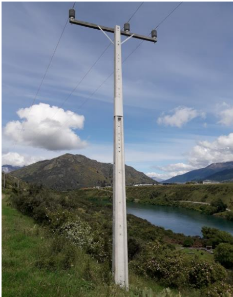
Figure 8.1: Example of a concrete pre-stressed pole
