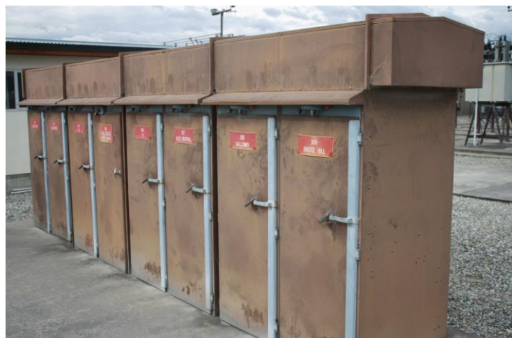
Figure 8.59: Indoor minimum oil-filled circuit breakers (left) installed in 'outdoor cubicles' (right)
