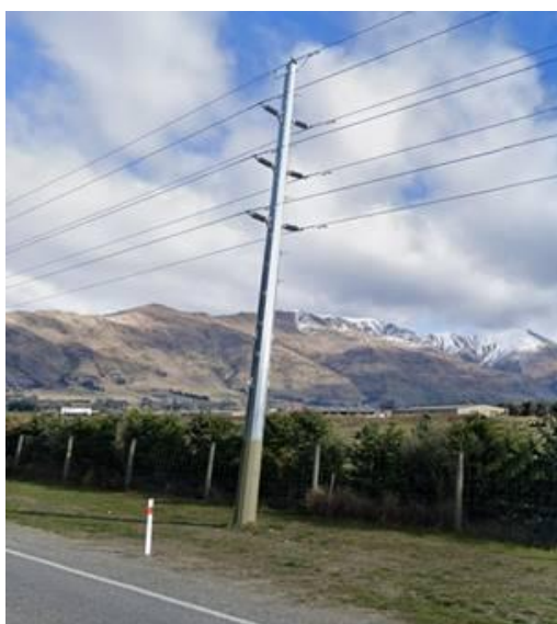
Figure 8.2: Example of a steel pole
