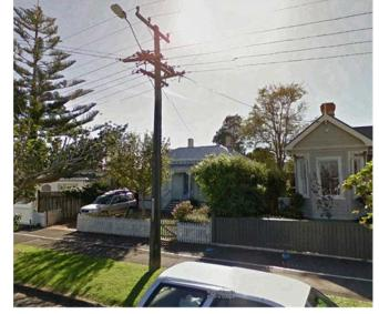
This example photograph shows a very congested pole. The lines company required the street lamp to be relocated, at Chorus' cost, before the pole could be used for aerial fibre deployment.
