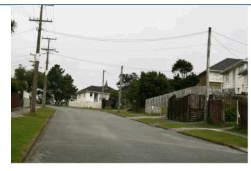
In this photograph, the poles on the right hand side are Chorus-owned. They would require strengthening or replacement to carry electricity lines (other than lead-ins). As such, Chorus could not offer to share them with a lines company. An HEO would encounter the same issue, unless it installed stronger poles (at a correspondingly higher cost).
