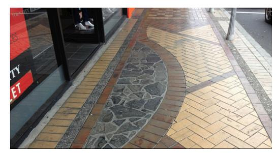
Figure C7: "like for like" reinstatement of specialty paving.
