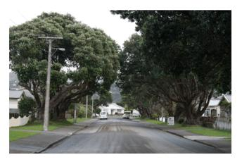
In this example, aerial deployment would be possible but not straight forward. Negotiating the trees will add to cost (and here, the tree interference is in the cable span and not around the pole heads). An HEO may well find it is cheaper to deploy underground, assuming that can be achieved under RMA consent conditions and without damaging tree roots.
