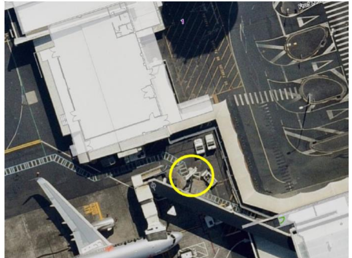
Image of where the unused bridge structure is currently located. (Gate 20 to bus lounge)
