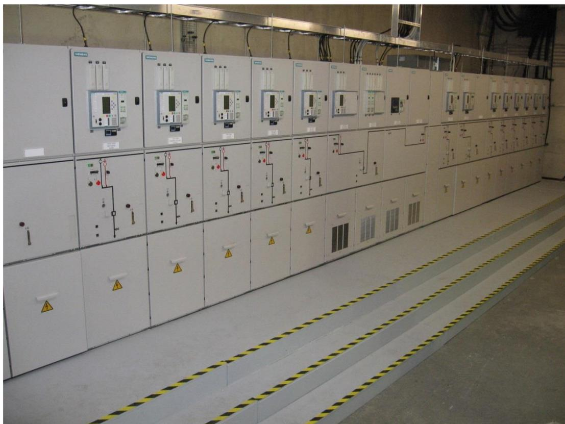
Photo of an 11 kV Circuit Breakers at The Terrace Zone Substation
