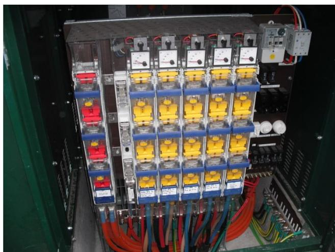
Photo of Low Voltage Disconnect Switches/Fuses
