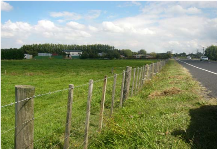
Fig 2 – Wooden post and batten 6 wires + 1 barbed wire fence
