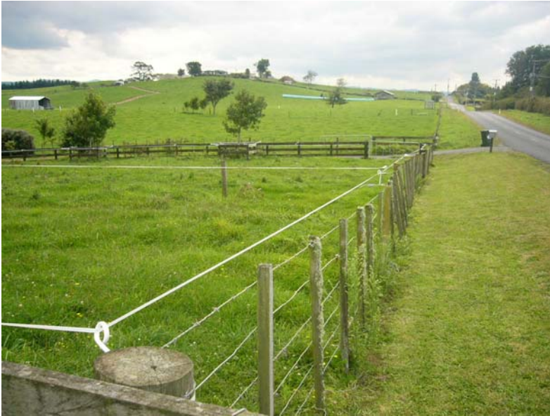
Fig 8 – Combination – Wooden post and batten fence with pigtail offsets and electrified tape
