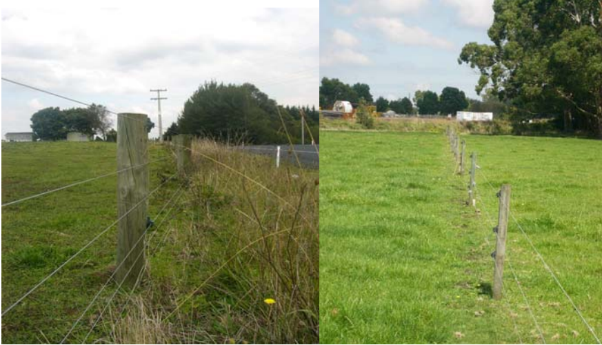
Fig 4 – Wooden post and fabricated wire fence and one barbed wire
