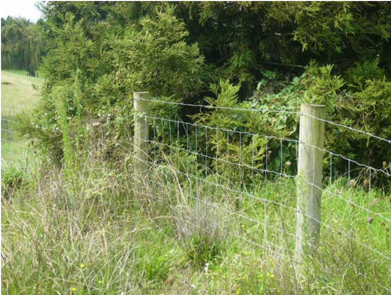
Fig 4 – Wooden post and fabricated wire fence and one barbed wire
