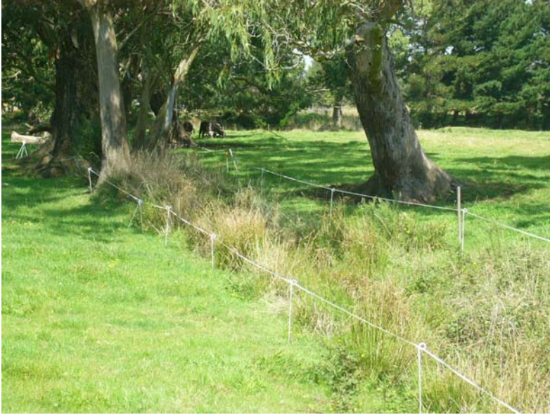
Fig 8 – Combination – Wooden post and batten fence with pigtail offsets and electrified tape
