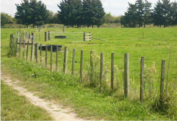
Fig 1 – Wooden post and batten 6 wire fence
