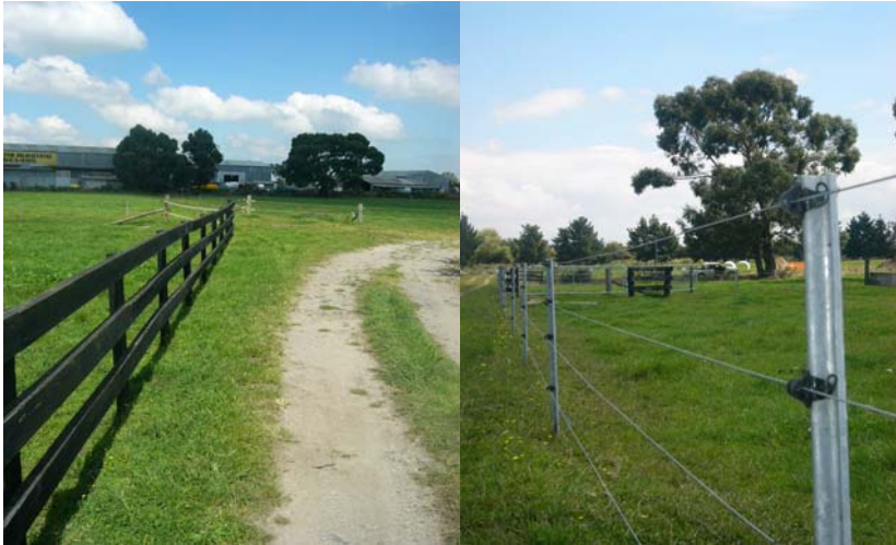
Fig 6 – Self Insulating (‘Gallagher Insultimber’) Post and three wire electric
