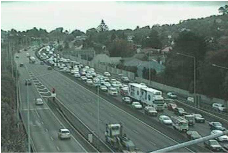
The Southern Motorway at Greenlane Rd (NZTA)
