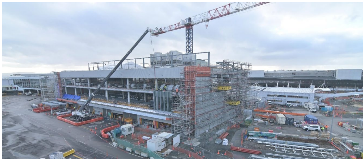
Figure 9: Construction of East Terminal Enabling project, July 2024
