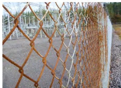
Figure 45: Example of Buildings and Grounds issue: deteriorating mesh
