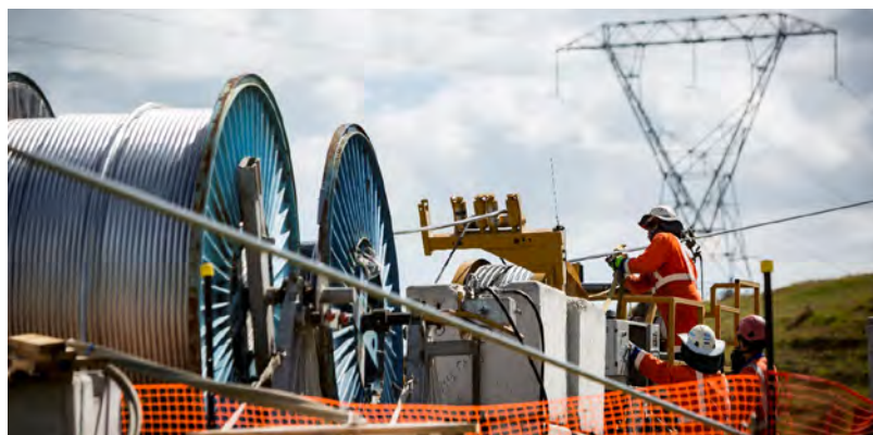
Figure 26: Reconductoring in progress
