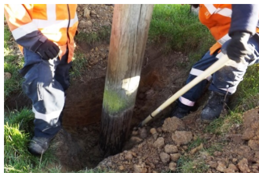
Pole base inspection – hand digging last part
