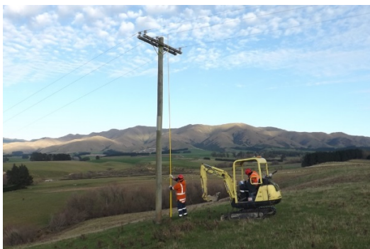
Checking pole and conductor height
