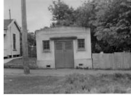
Bronte Street substation 1950 – still in use today
