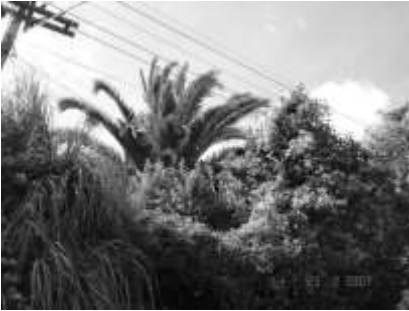
Trees close to powerlines Feb 2007
