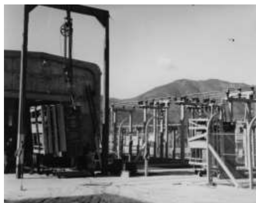
NEL's 33kV transformers arriving in Jan 1960
