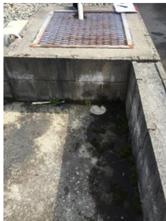
Photo 5: Fernhill ZSS: subject to verification, bund drainage from T1 looked to flow into T2 bund using a PVC drainage pipe; non fire retardant, no flame trap. Tee joint in T2 bund, connection T1 and the drainage sump
