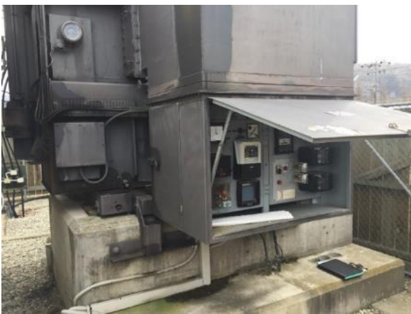
Photo 3: Clyde Earnsclough ZSS – non-functioning protection relay (one phase) on right hand side of cabinet
