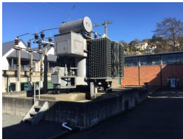
Photo 5: Fernhill ZSS: subject to verification, bund drainage from T1 looked to flow into T2 bund using a PVC drainage pipe; non fire retardant, no flame trap. Tee joint in T2 bund, connection T1 and the drainage sump
