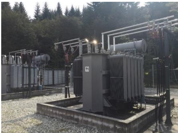
Photo 5: Fernhill ZSS: subject to verification, bund drainage from T1 looked to flow into T2 bund using a PVC drainage pipe; non fire retardant, no flame trap. Tee joint in T2 bund, connection T1 and the drainage sump
