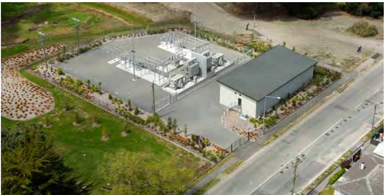
Our Keys Road substation was quickly built after the February 2011 earthquake.
