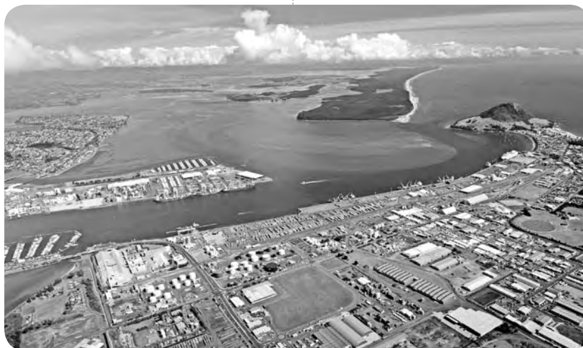
Port of Tauranga. Photo: Port of Tauranga Ltd.
