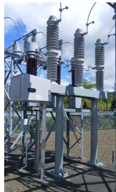
Figure 18.12: Live tank SF 6 outdoor 33kV circuit breaker
