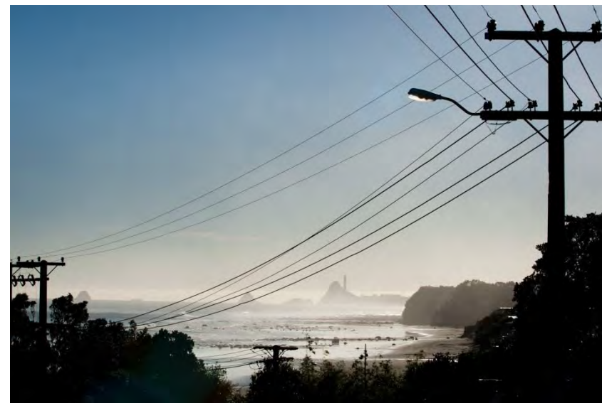
Figure 16.6: Distribution overhead line with LV underbuilt
