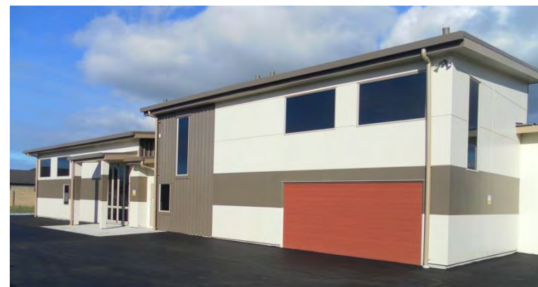
Figure 18.15: Urban zone substation building
