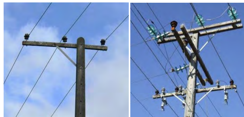
Figure 15.8: Different crossarm configurations
