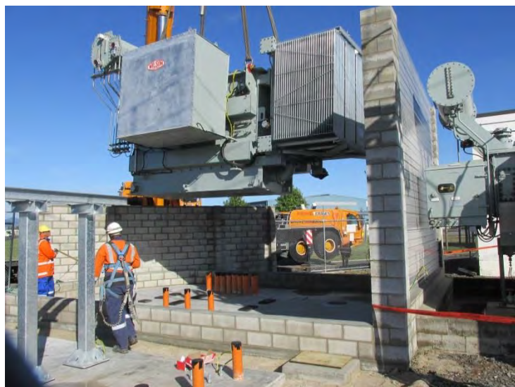
Figure 18.1: Power transformer installation at Waharoa
