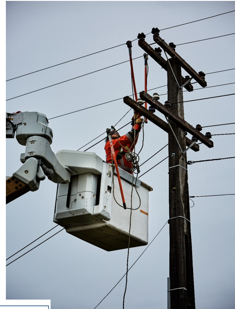
Figure 12: Field technician working at height on overhead asset de-energised
