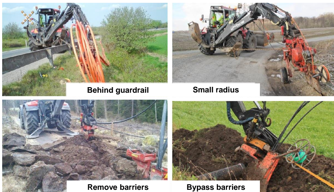
Figure 2-7: Flexible trenching tools improve efficiency significantly
