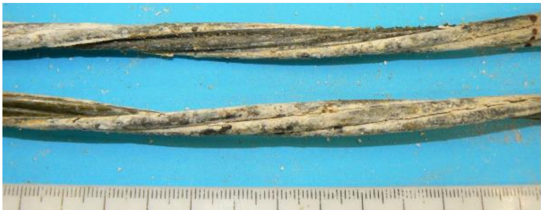
Figure 8 - Steel core wires as identified in Figure 5, note the dried grease and corrosion product on the wires.
