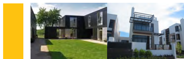
Detached single family dwellings within Seatoun-style neighbourhoods offering flat sections, offstreet parking and easy walk to foreshore and town centre
