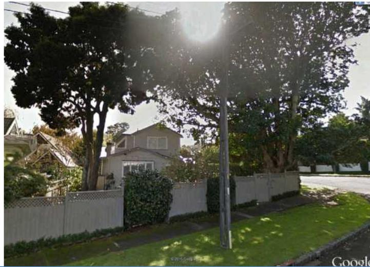
In this photograph, the pole was assessed as requiring replacement because it was not sufficiently robust to support additional aerial fibre lines.
