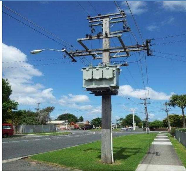
This example photograph shows multiple voltage lines and the placement of a transformer and a street lamp on a pole. Deployment on this pole would involve significant rearrangement, possible strengthening, and onerous HSE requirements given the electricity lines all around the pole. Such severe congestion means that Chorus (or the HEO, as applicable) is unlikely to be able to use this pole for aerial fibre deployment.
