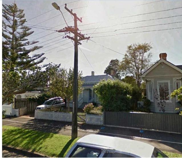
This example photograph shows a very congested pole. The lines company required the street lamp to be relocated, at Chorus' cost, before the pole could be used for aerial fibre deployment.
